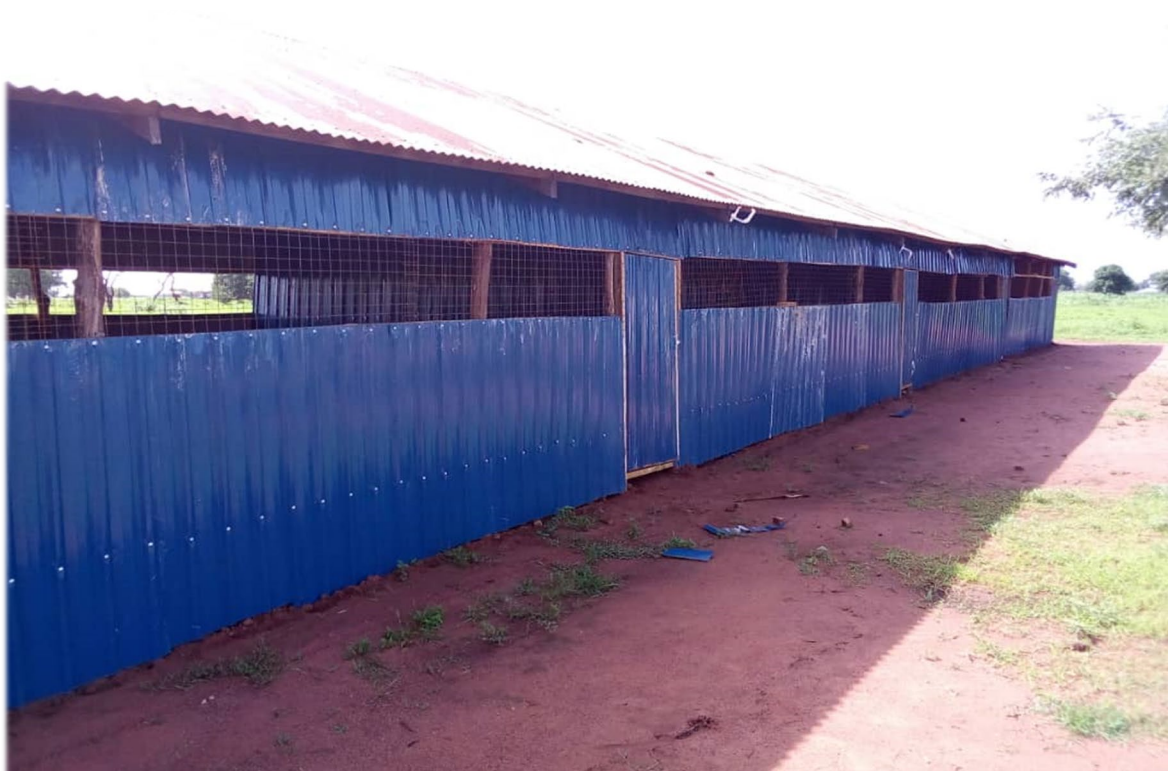
Three classrooms temporary learning spaces constructed by WTI
