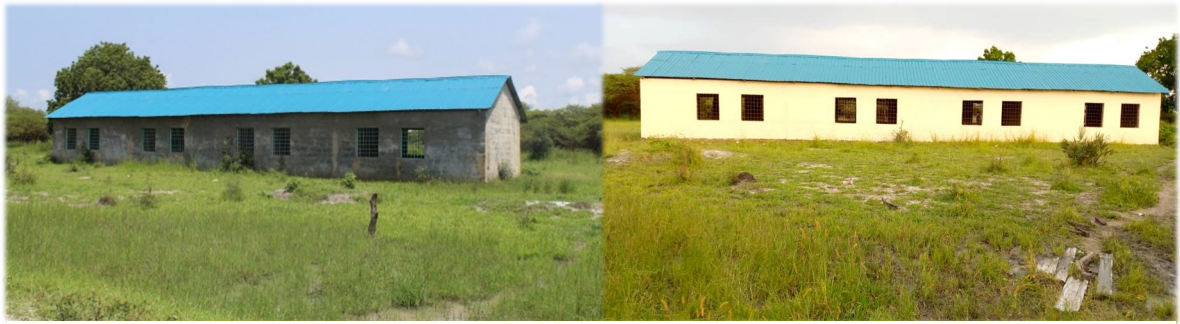
Two classroom block renovations: before and after
